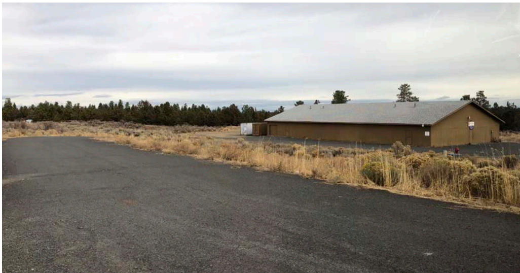
CNG odorizing facility on Knott Road
